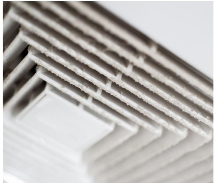
ing in the first place by minimizing dirt, debris, and microbiological growth in the system, maintaining filter systems and using filters rated at MERV 7 or greater, and conducting regular HVAC inspection and maintenance.
